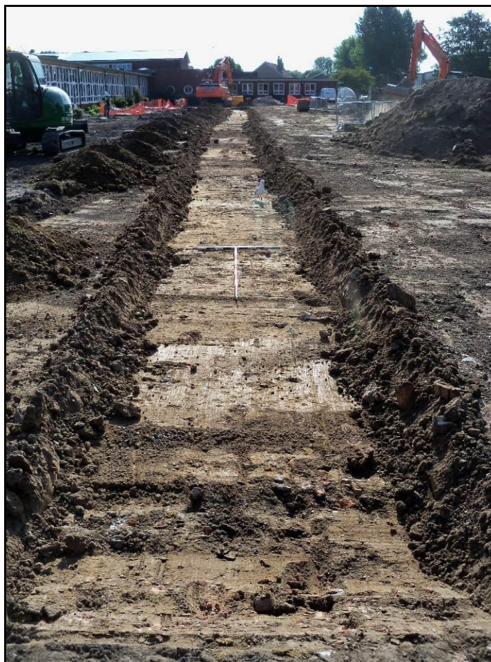
Plate 1: Highfield Junior School, Eastbourne: Trench 1 looking east
