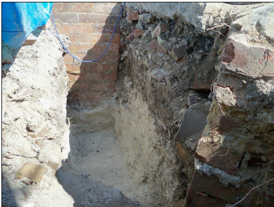
Fig. 6: 202 Willingdon Road, Eastbourne: Photograph of trench section
