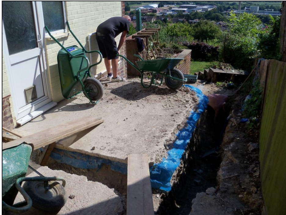
Fig. 5: 202 Willingdon Road, Eastbourne: Photograph of site
