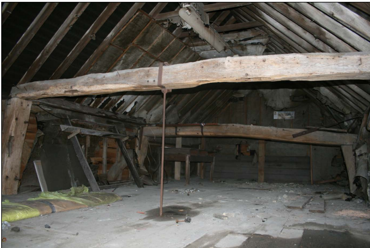
Fig. 13: Crown View, Horsted Keynes: First floor roof space
