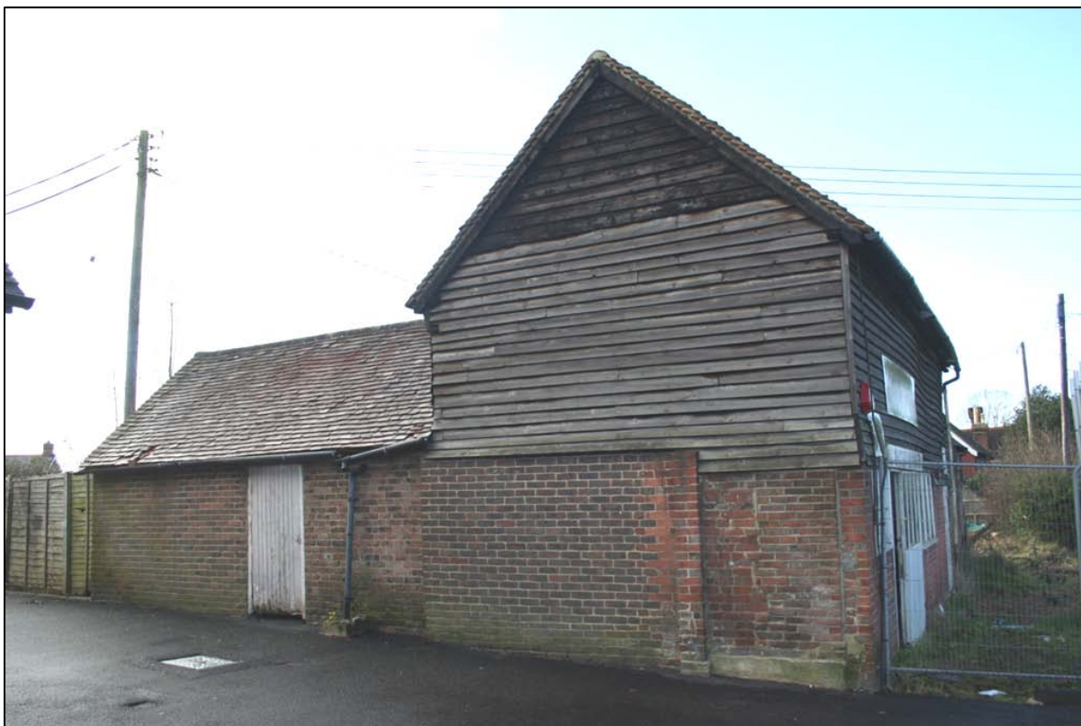
Fig. 12: Crown View, Horsted Keynes: External view of east wall
