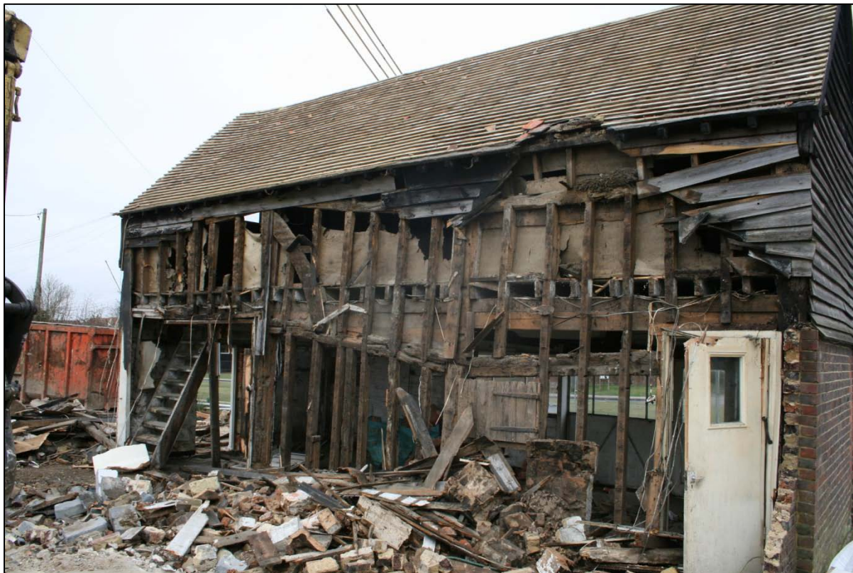
Fig. 15: Crown View, Horsted Keynes: External view of south wall during demolition
