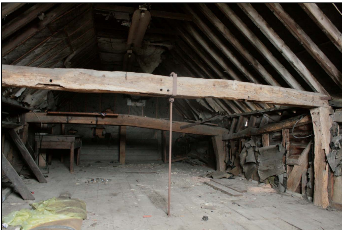
Fig. 14: Crown View, Horsted Keynes: First floor roof space
