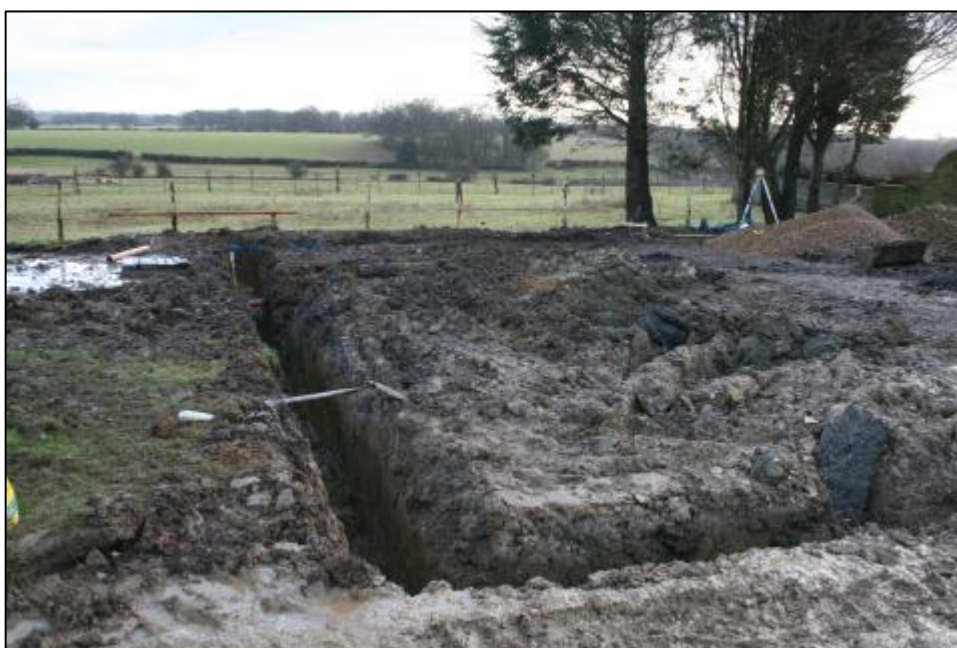
Fig. 8: Methersham Farm, Beckley: Photograph showing excavation of footings
