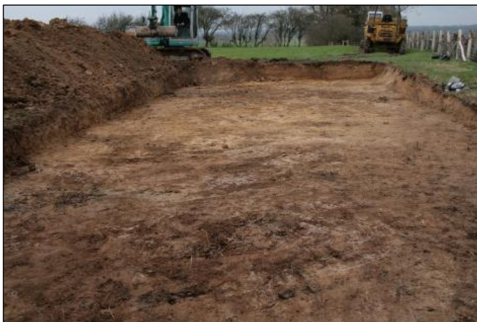
Fig. 7: Methersham Farm, Beckley: Photograph showing reduction over new site of stables
