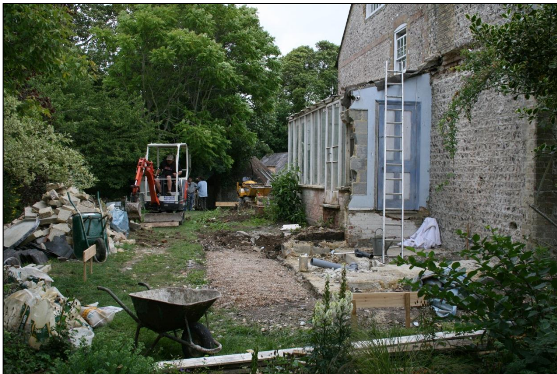
Fig. 6: Grange Farm, South Heighton: Photograph of site
