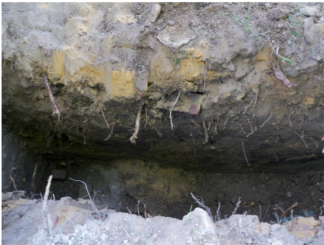
Fig. 5: North Lodge, Mayfield: Photograph of footing trench showing mixed nature of topsoil/made ground
