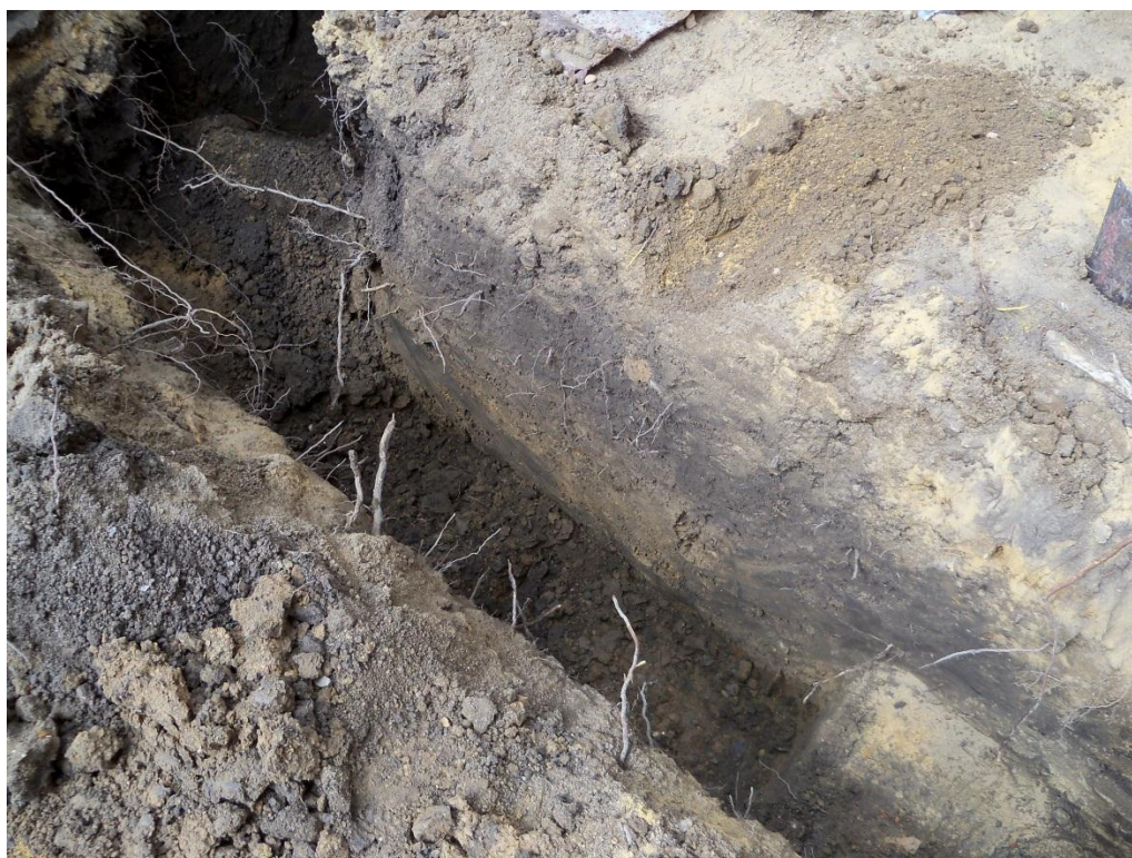
Fig. 6: North Lodge, Mayfield: Photograph of footing trench showing stratigraphy
