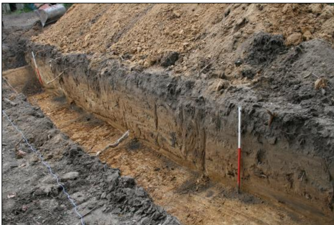
Fig. 12: Trench B Photograph
