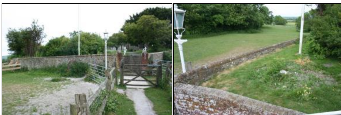
Plate 1: Alciston Church: The site prior to work commencing
