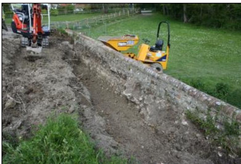
Plate 3: Alciston Church: Excavation for the French Drain
