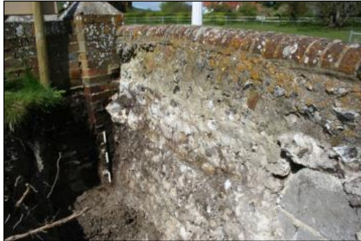
Plate 4: Alciston Church: Different phases of wall construction
