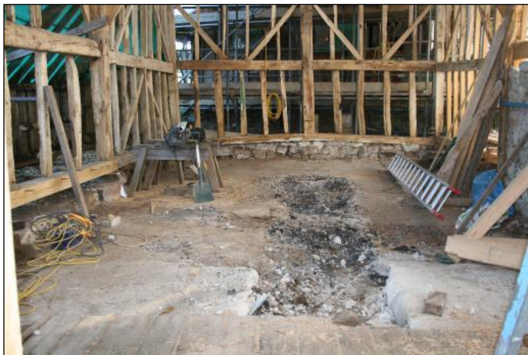
Plate 1: Trench A and the east end of the Barn
