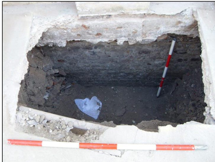
Plate 3: Infilled brick built cellar
