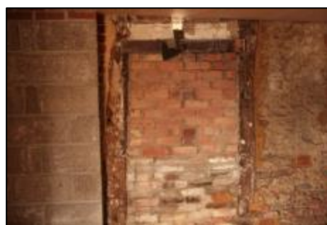
Plate 17: Possible Doorway in Northern Wall of Bay 4
