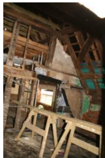
Plate 26: South End of West Wall Bay 2
