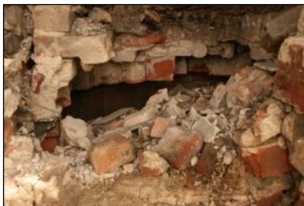
Plate 10: Structure to South of the Inglenook from Exterior
