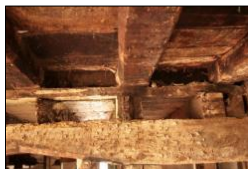
Plate 14: Joists of Bay 2 and Bay 3
