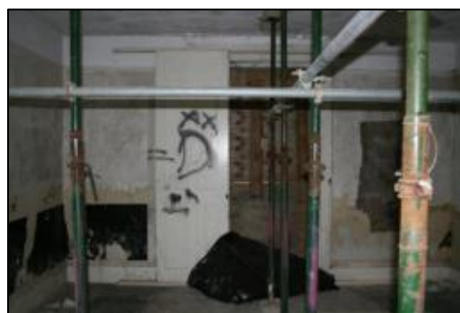
Plate 36: Example of Sliding Shutters
