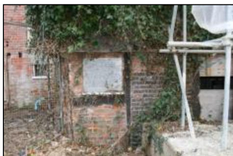
Plate 3: Framing in North end of West Wall
