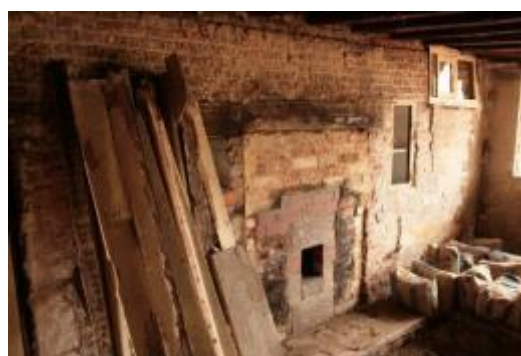
Plate 9: Second Cupboard with Area of Repair Below
