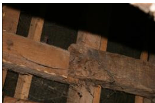
Plate 32: Joint in Purlin North Side Bay 1
