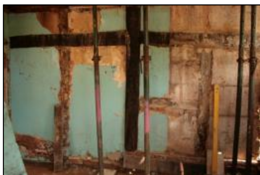
Plate 6: Framing in North Wall of Kitchen
