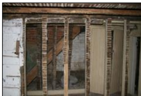
Plate 16: Northern Stud Walls of Staircase and Corridor
