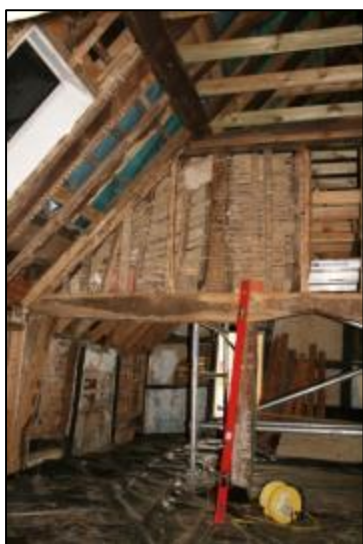
Plate 25: North End of West Wall Bay 2
