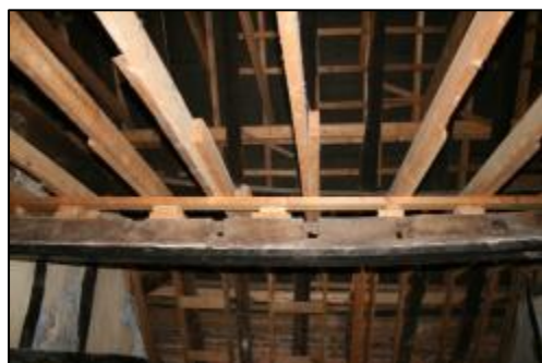
Plate 23: Ceiling Girder in Bay 3
