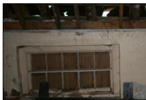
Plate 2: Example of first Floor Window
