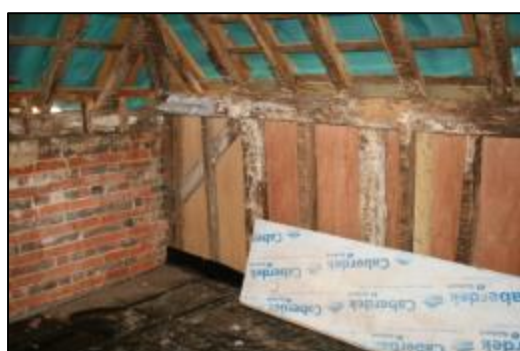
Plate 28: South End of West Wall Bay 1
