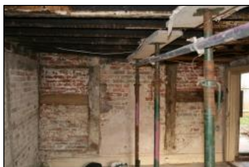
Plate 13: North Wall of Bay 3
