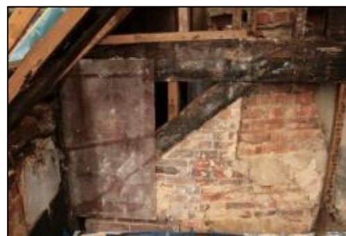
Plate 19: Downward Brace in Bay 4
