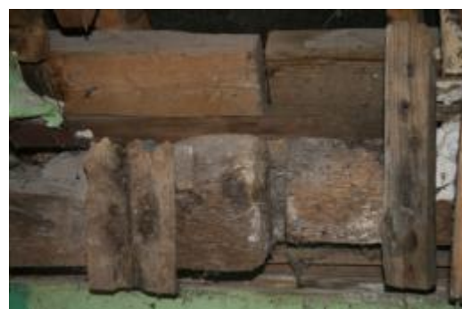
Plate 31: Joint in Southern Wall Plate Bay 1
