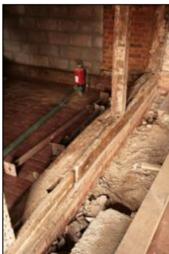
Plate 11: West Wall of Bay 3
