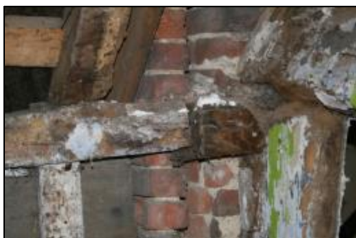
Plate 30: Joint in Northern Wall Plate Bay 1
