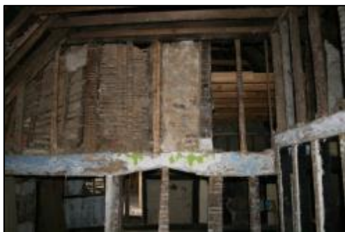
Plate 20: Door Head Between Bays 2 and 3
