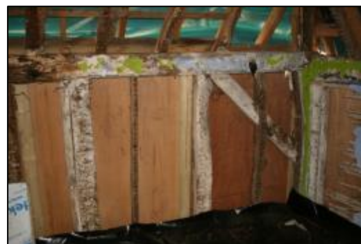
Plate 29: North End of West Wall Bay 1
