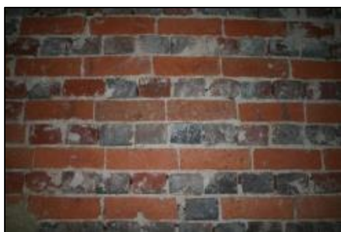
Plate 1: Interior brickwork Southern Wall
