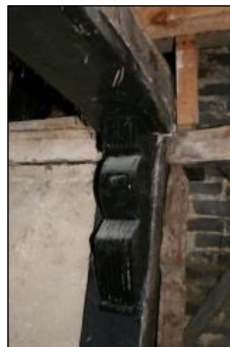
Plate 24: Ceiling Girder Corbel
