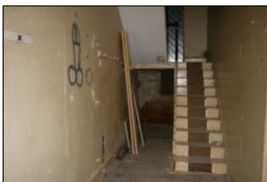
Plate 34: Corridor in 19 th Century Extension
