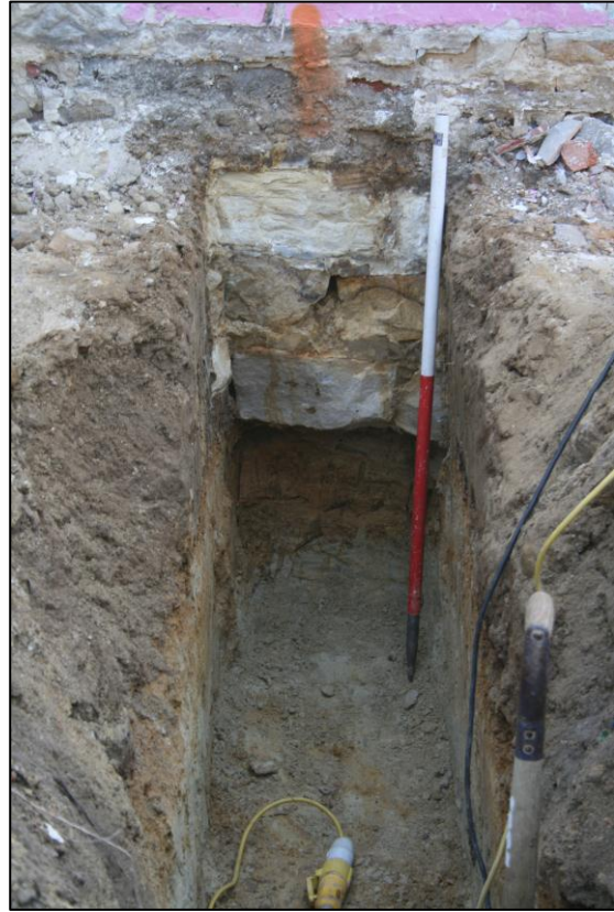
Fig. 8: Ore Place Farmhouse: Foundations of Farmhouse
