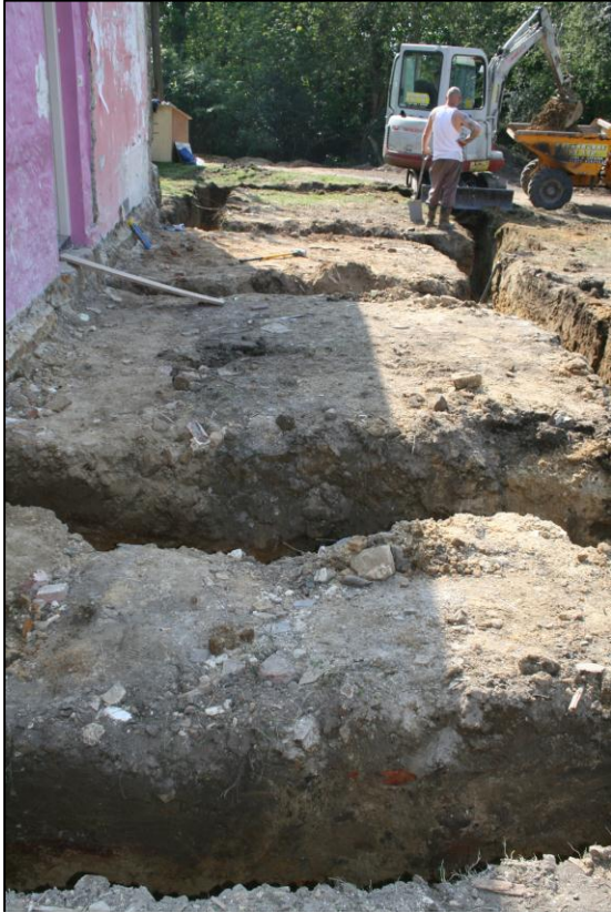
Fig. 7: Ore Place Farmhouse: Excavated foundations for new
