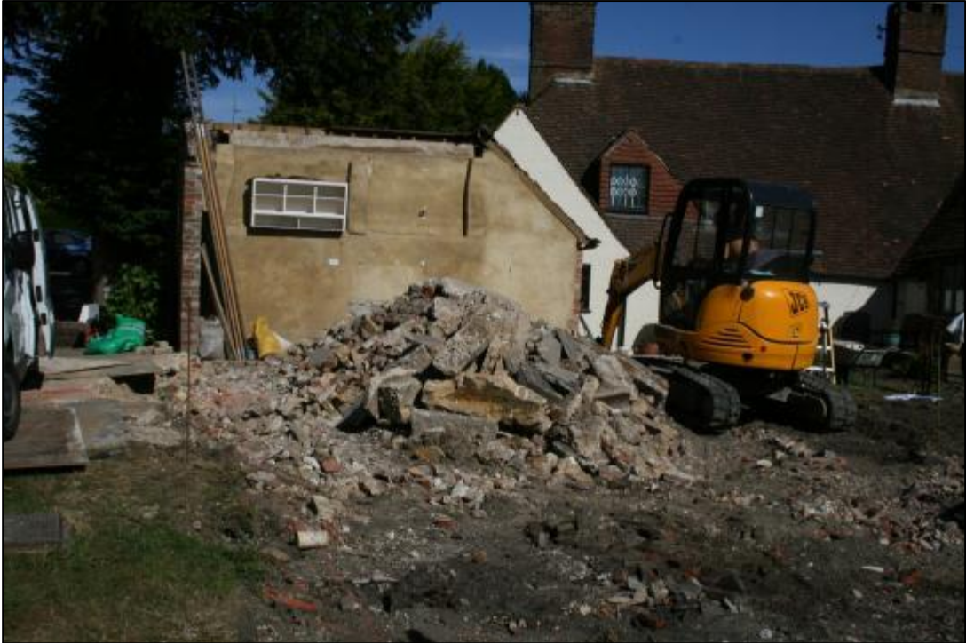
Fig. 7: The Yews, Lewes Road, Ringmer: General view of site
