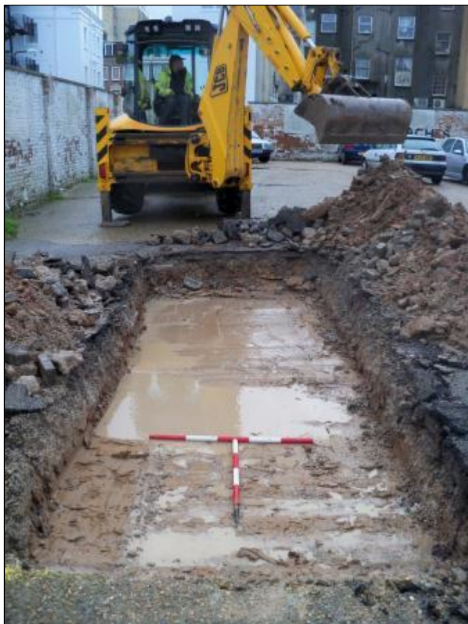
Plate 9: Burlington Hotel, Eastbourne: Trench 4; looking southwest
