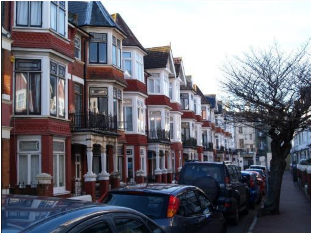
Plate 1: Burlington Hotel, Eastbourne: The front of the terrace on Elms Avenue, built c.1901, showing a consistent line of buildings with no indication of rebuilding; looking west
