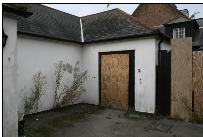
Plate 5: Storeroom at the western end of northern elevation
