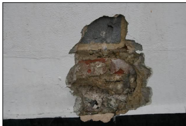
Plate 4: The two areas where the cement render had been removed.
