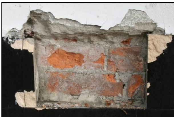
Plate 4: The two areas where the cement render had been removed.
