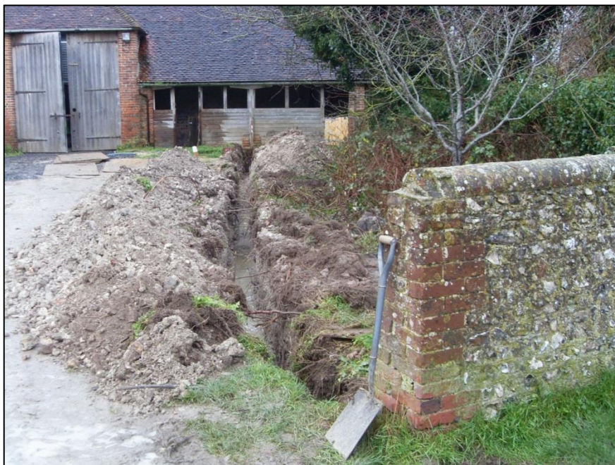
Plate 1: Route of service trench.
