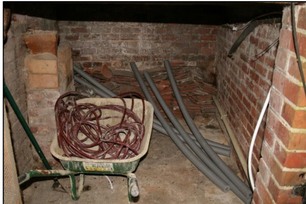
Plate 3: Building A store room
