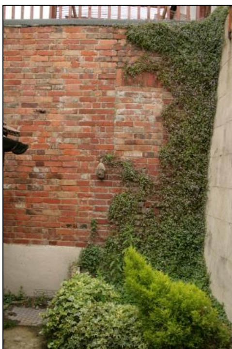
Plate 1: North Wall of Sunken Courtyard with Blocked Window at Eastern End
