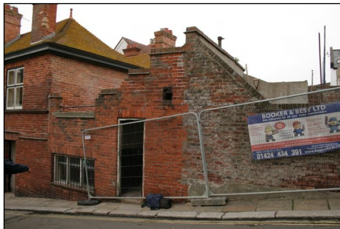
Plate 4: Southern Elevation of the Buildings from Crown Lane
