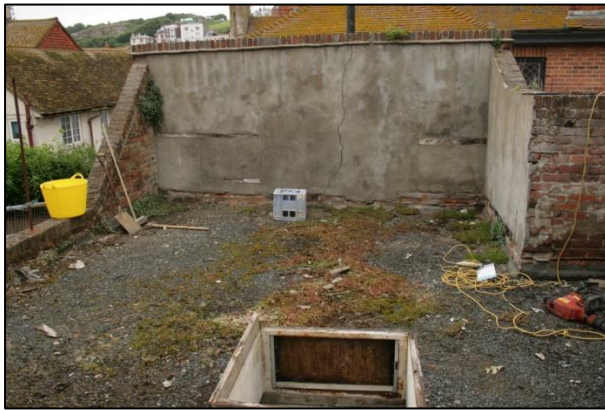
Plate 9: Western Enclosing Wall of the Roof to Building B
