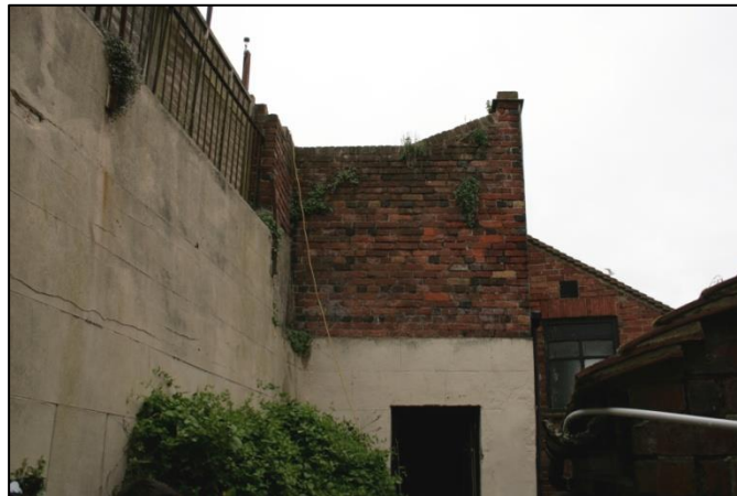
Plate 5: Northern Elevation of Building B
