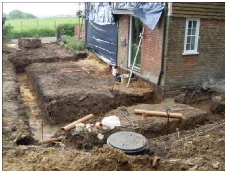
Plate 1: Excavated footing trenches
