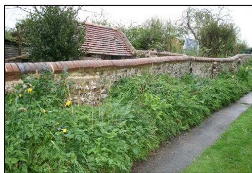
Plate 4: Buttresses at North-western end of the Wall
