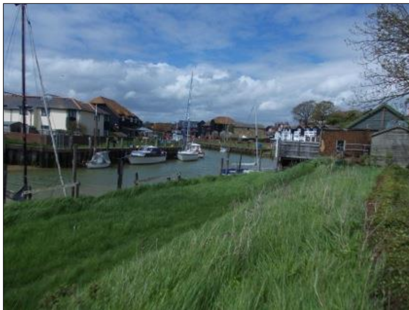
Plate 5: Sea defences and moorings behind the Site with the former warehouses of the quayside in the background, looking north
