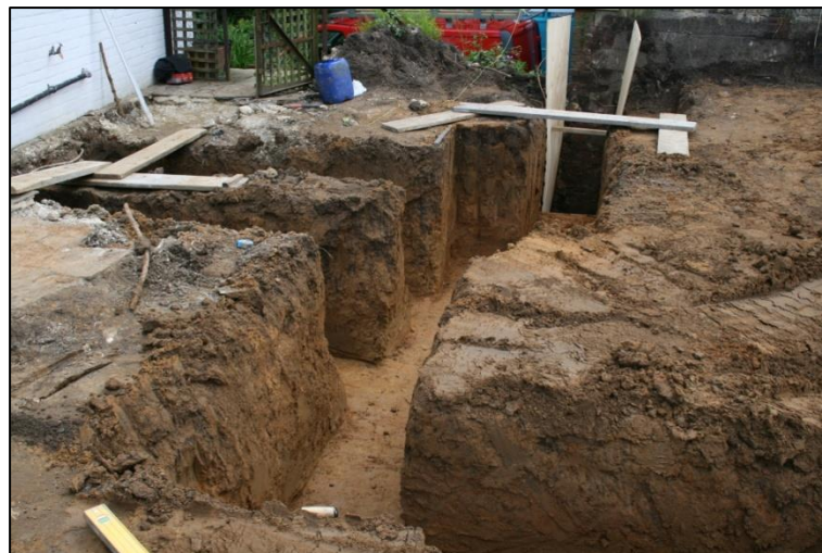
Plate 3 White Hart Cottage: The completed footings trenches
