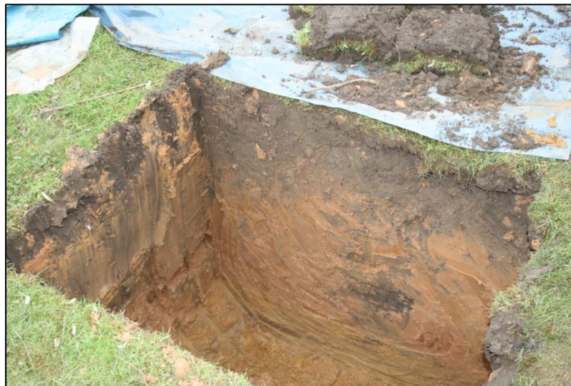
Plate 4 White Hart Cottage: Trench for soak-away
