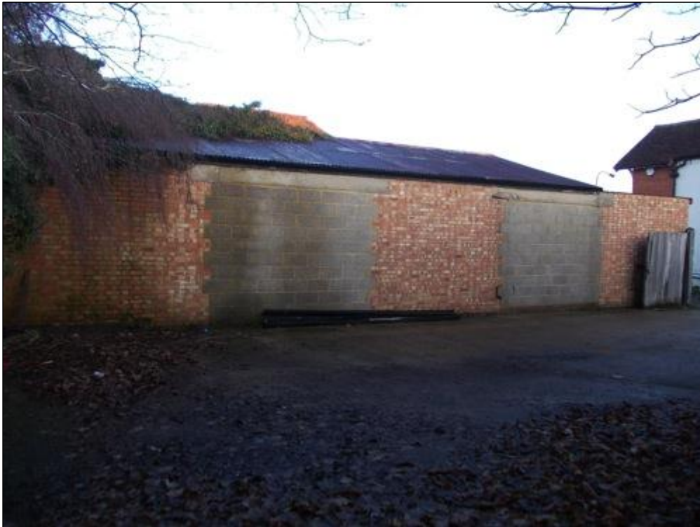
Plate 5: Buildings 6 and 7, looking northeast
