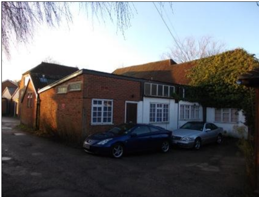
Plate 1: Barn 1 and Buildings 3 and 4, looking southwest
