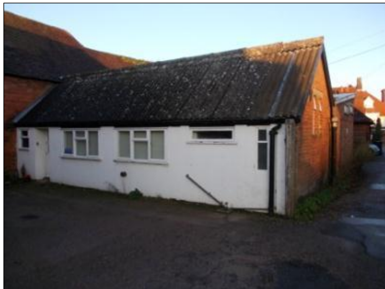
Plate 3: Building 4, looking northwest
