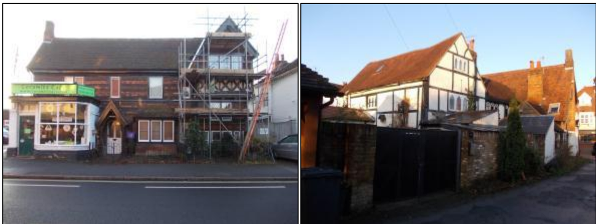
Plate 6: Front and back views of the adjacent Listed Building
