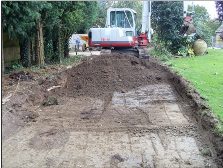
Plate 2: Phase 1 looking west
