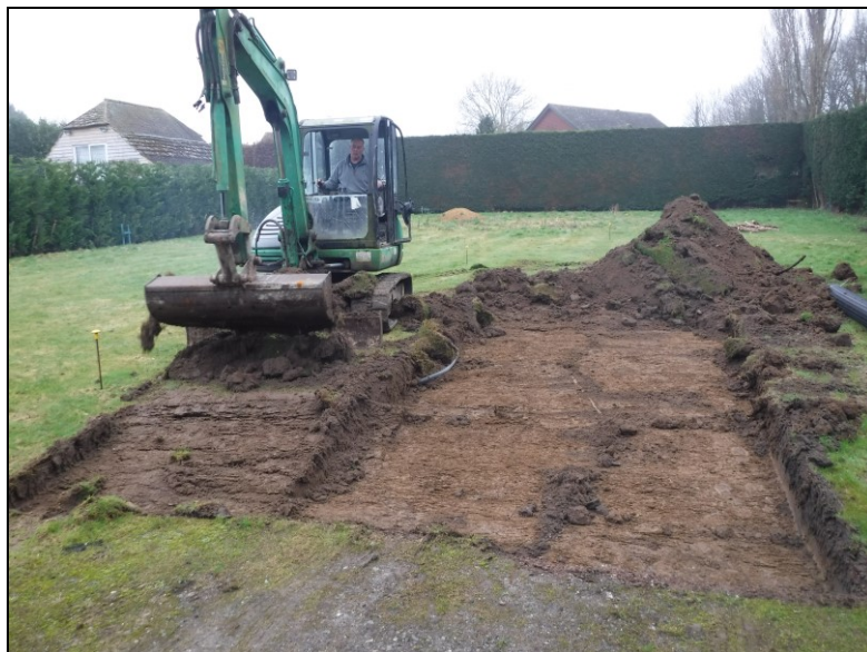
Plate 3: Phase 2 Working shot looking north
