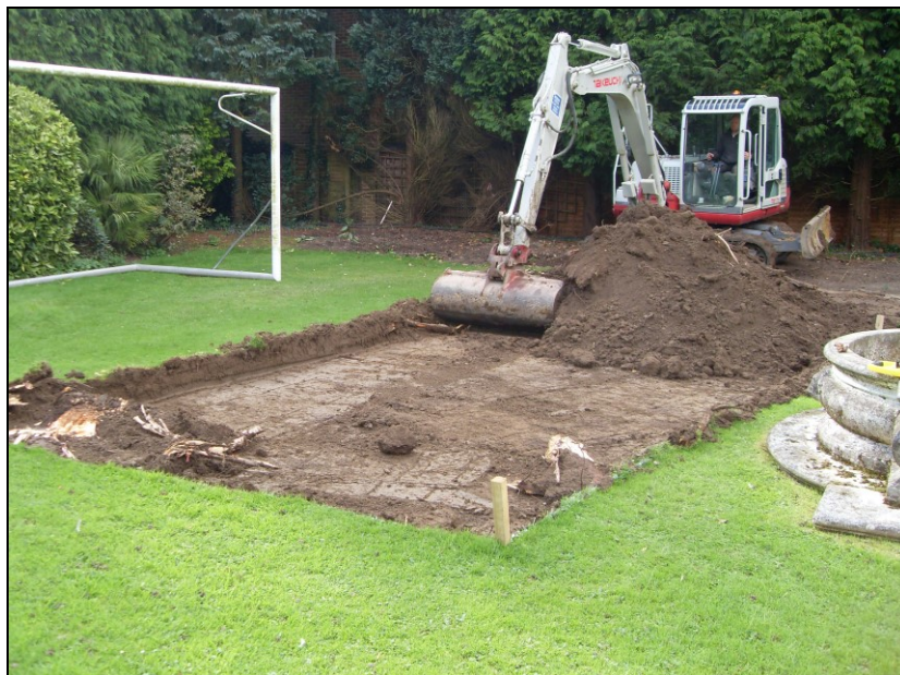
Plate 1: Initial Phase 1 of excavation looking south-west
