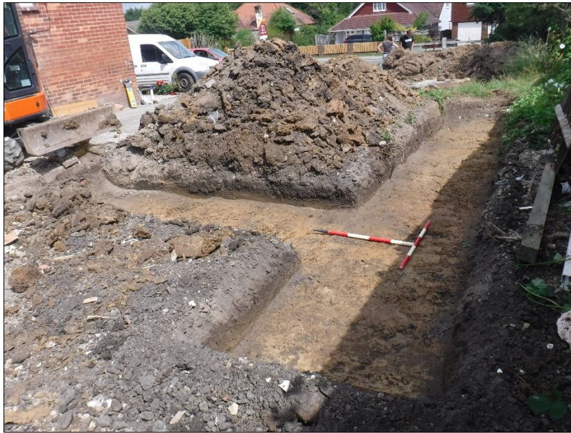
Plate 5: The Site looking northwest, showing Trenches 2 and 3
