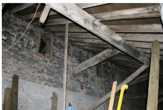
Plate 14: Dividing Wall East Side
