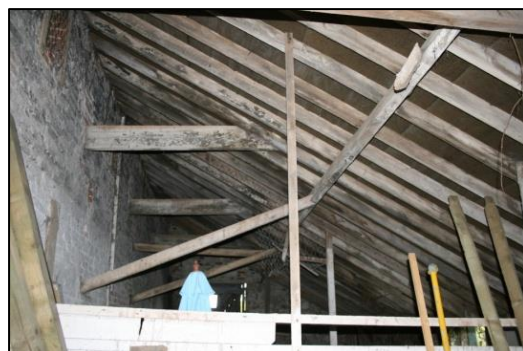
Plate 16: Construction of Stable Roof
