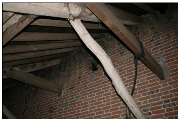
Plate 13: Roof Braces in Roof of Store
