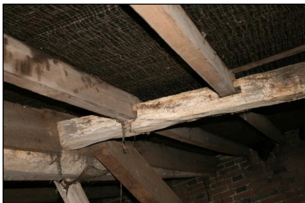
Plate 11: Earlier Mortises in Purlin
