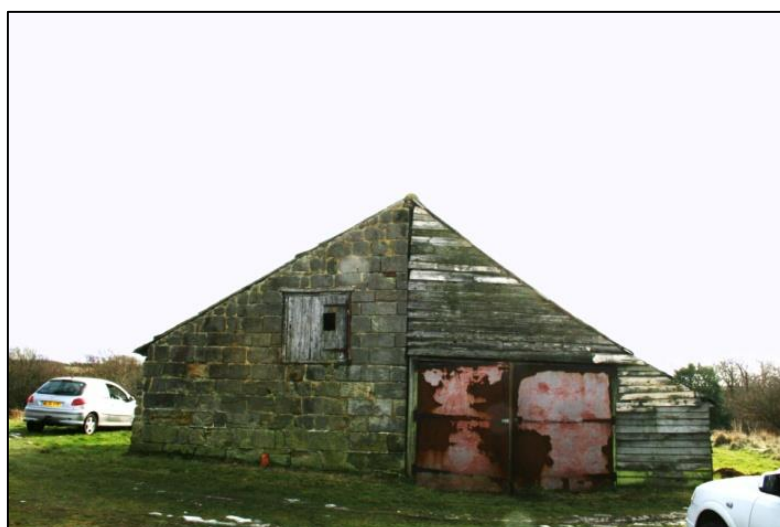
Plate 1: Northern Elevation of Barn
