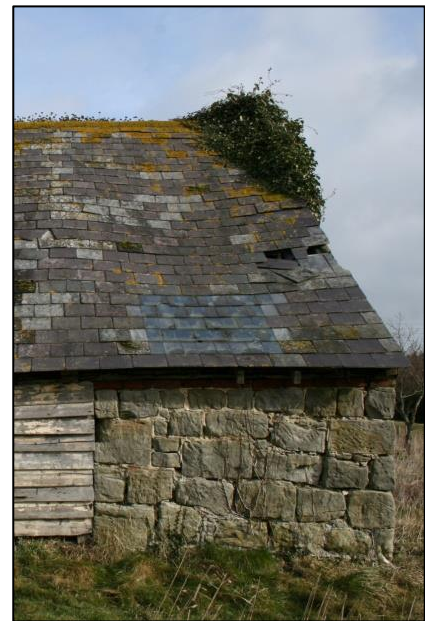
Plate 3: Sandstone Blocks at southern end of the West Wall
