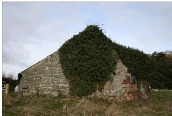
Plate 4: Southern Elevation of Barn
