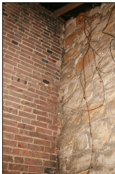
Plate 8: Southern End of Dividing wall
