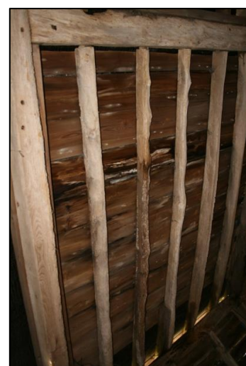
Plate 12: Original Rafters (Un-worked Timbers)
