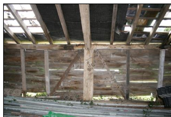
Plate 10: Low Posts and Studs of western wall
