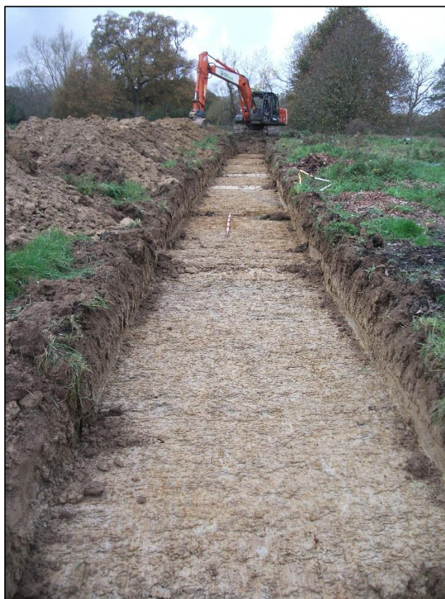
Plate 1: Initial trench excavated across the site
