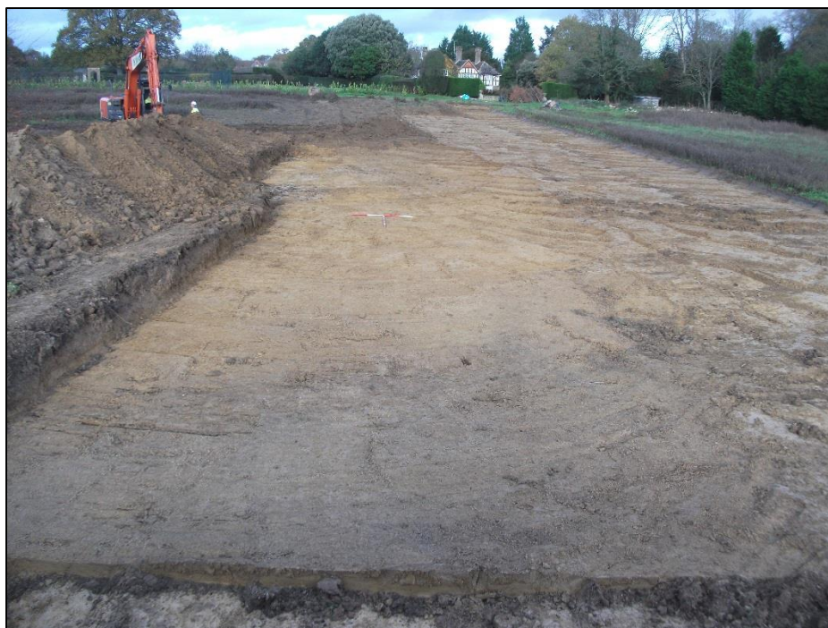
Plate 2: Part of site stripped of topsoil
