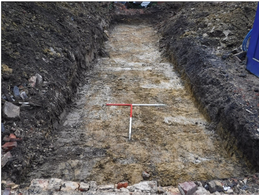
Plate 3: Trench 1, looking southeast
