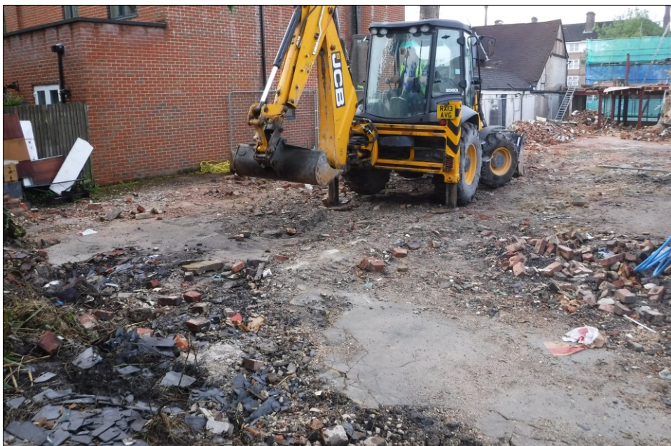
Plate 1: The Site prior to excavation, looking southeast
