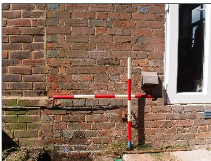
Plate 7: Brickwork detail of eastern elevation. Looking west. 1m scale.
