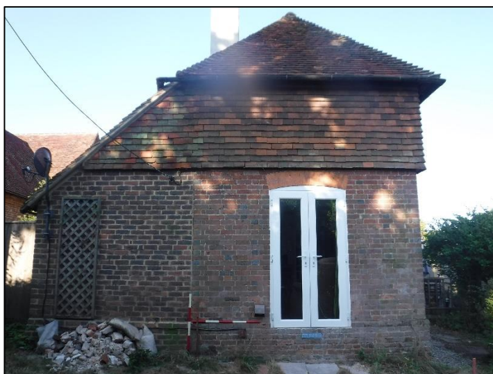
Plate 6: Eastern elevation of existing building. Looking west. 1m scale.
