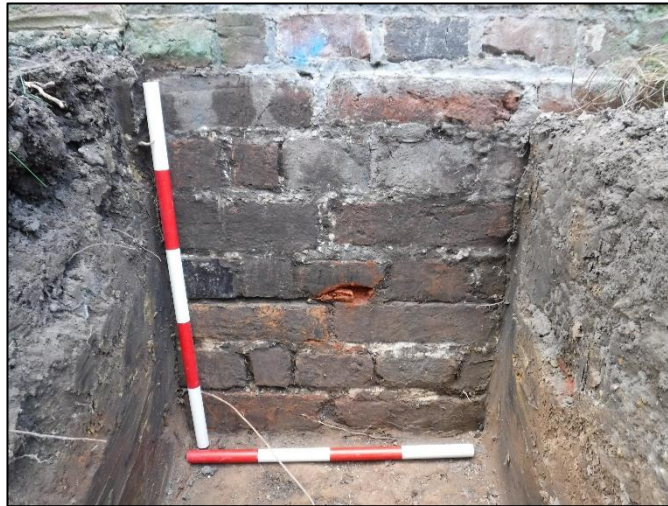
Plate 4: Exposed foundation (Context 004 ) of existing building
