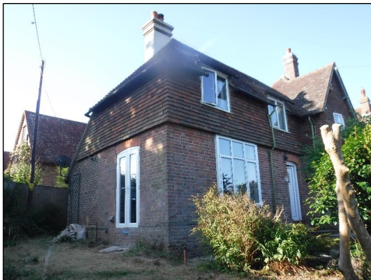
Plate 5: Eastern and northern elevations of existing building. Looking southwest.
