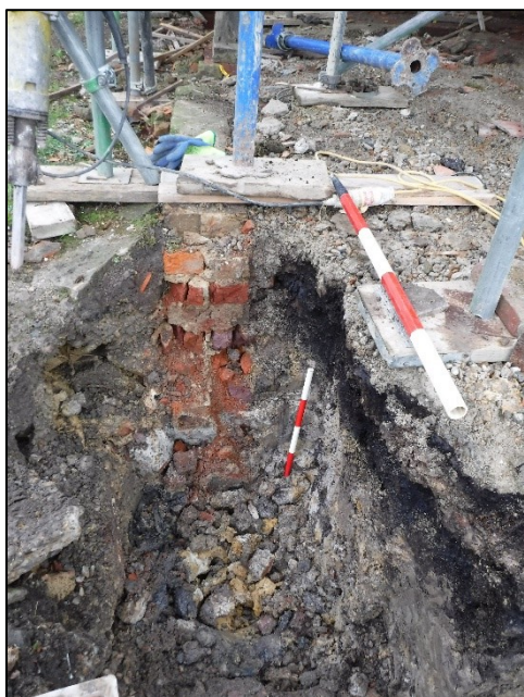
Plate 4: Barn foundation work
