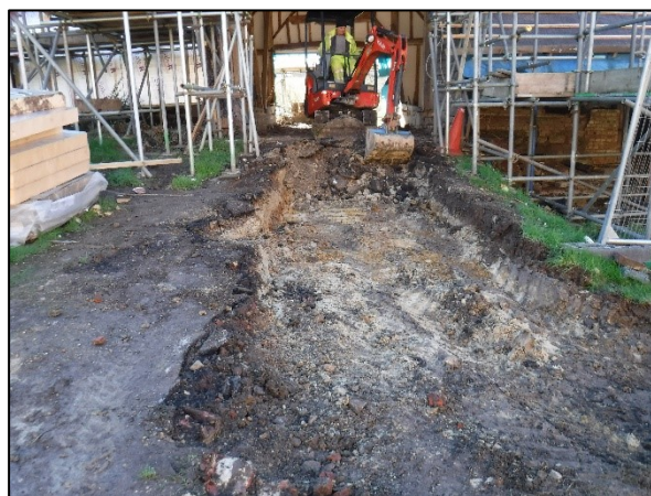
Plate 5: Lowering of ramp to barn
