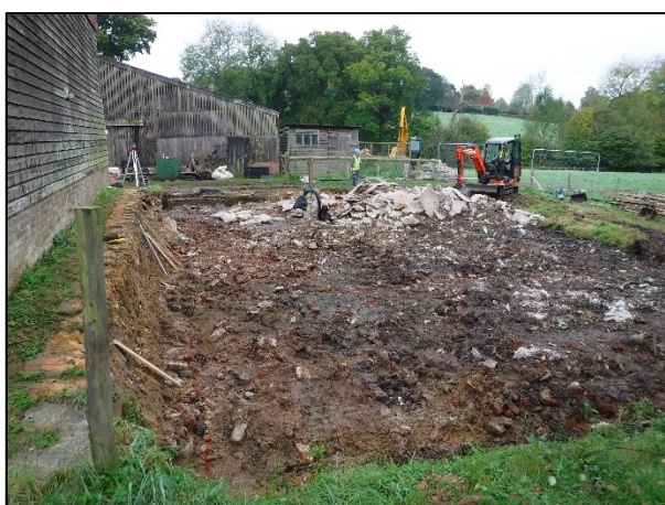
Plate 2: Brye after demolition
