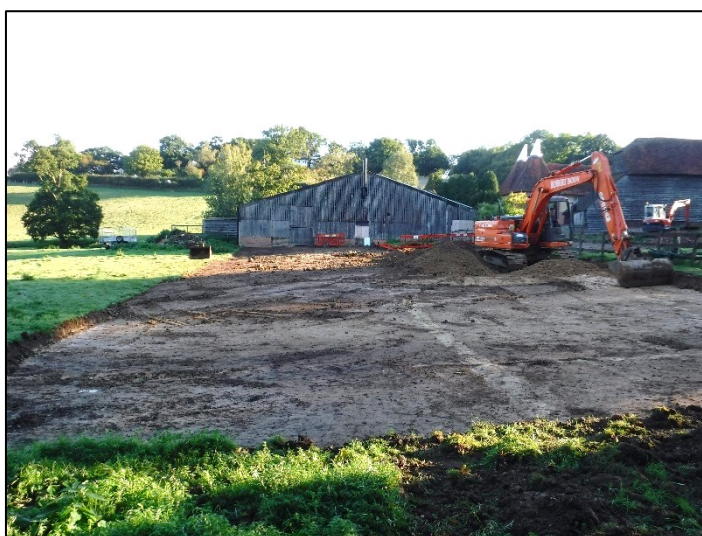
Plate 1: Ground reduction for car park
