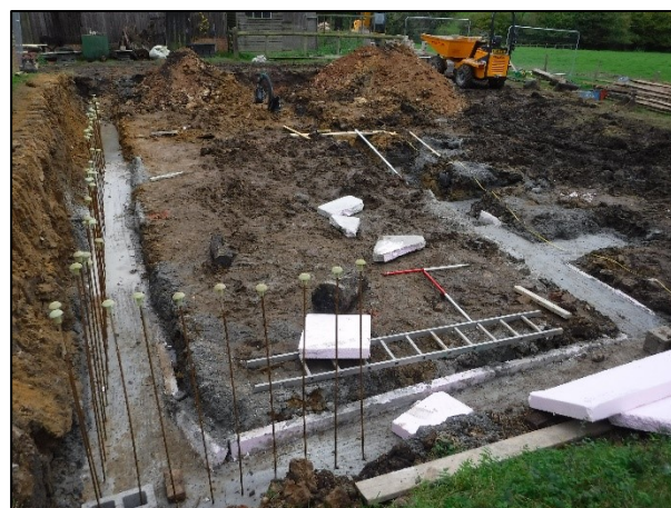
Plate 3: Excavation of foundation trenches
