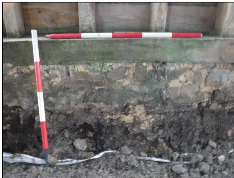
Plate 4: Surviving western elevation foundation at south end
