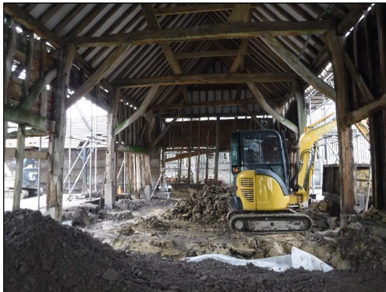
Plate 1: Working shot looking south in the barn
