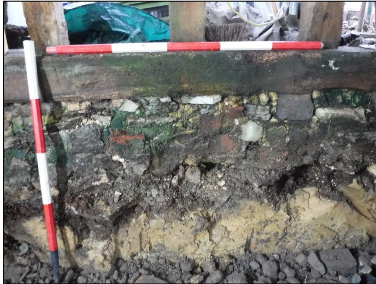
Plate 5: Northern and eastern elevation foundation
