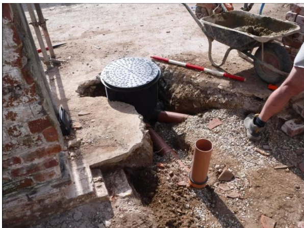
Plate 2: Manhole in east wall of parlour building, facing east
