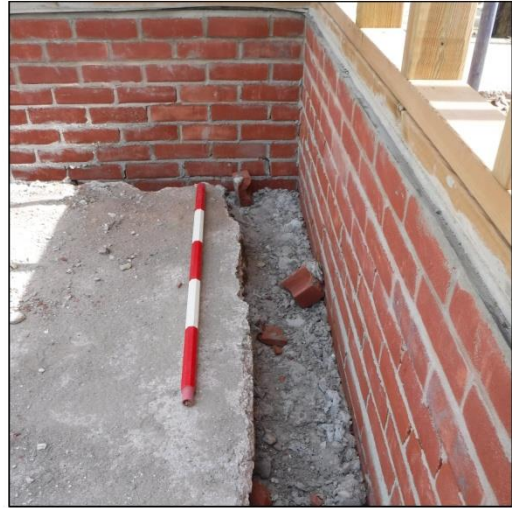
Plate 8: View of footings, northeast corner of the Store, facing north
