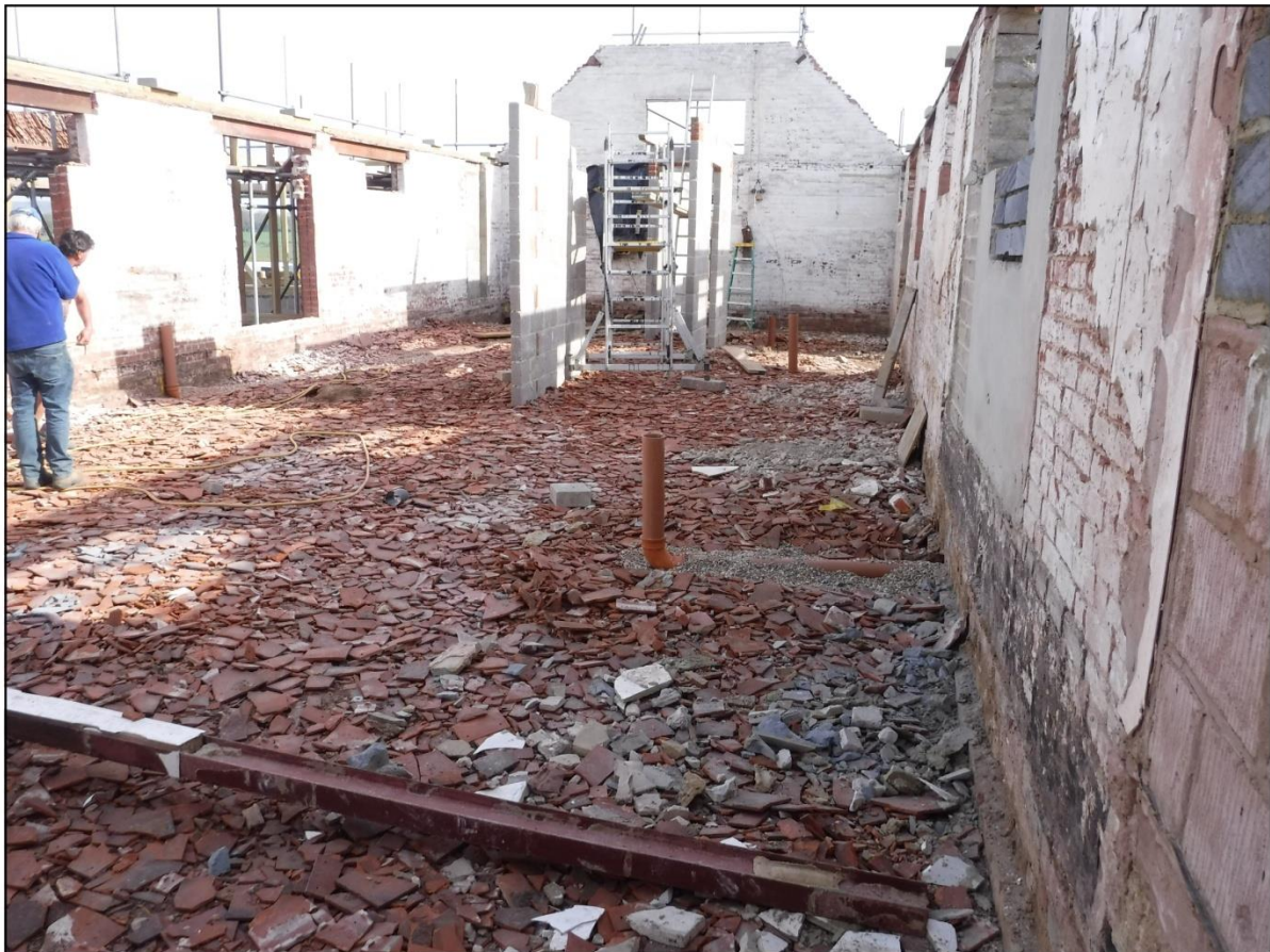
Plate 1: Internal view of the Parlour Building, facing north
