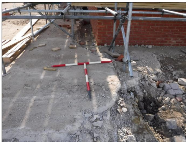
Plate 5: View of footings, northwest corner of Parlour extension, facing east
