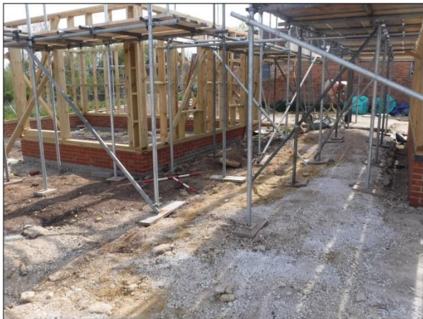
Plate 9: Southwest corner of the Stables’ east wing, facing east
