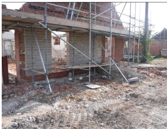
Plate 4: South wall of the Parlour, facing northeast
