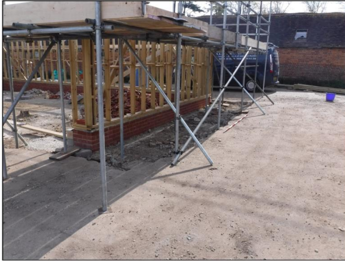
Plate 7: Southwest corner of the Store, facing east
