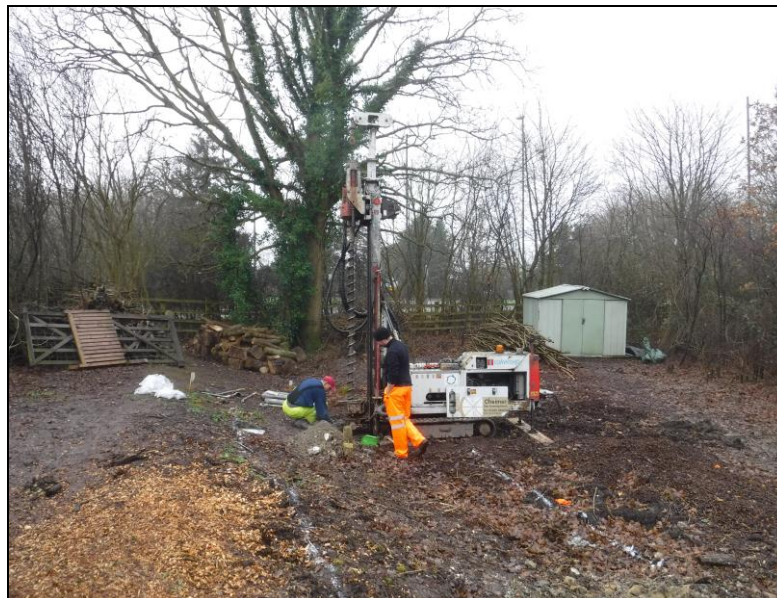
Plate 1: Location of second borehole looking south-west.
