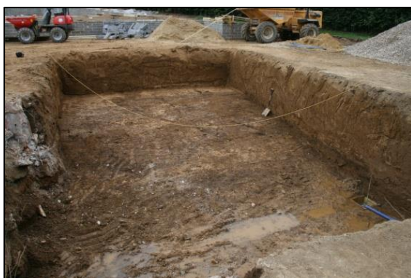
Plate 5: Trench for the new Swimming Pool
