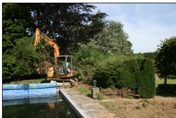
Plate 2: The grubbing-out of the Hedge to the north-west of Site
