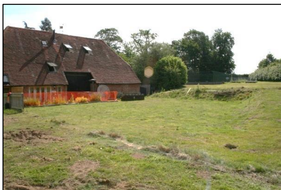
Plate 3: Converted Barn with Bank to the south-west
