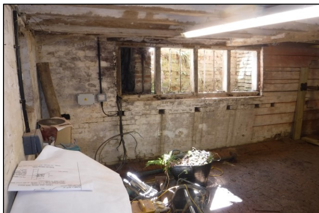
East wall of Cellar
