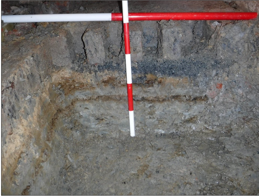
Plate 6: SW-facing section of Foundation Pit 5
