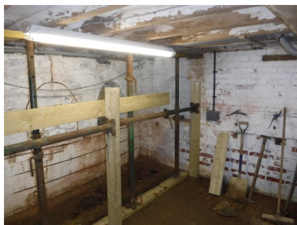
South-west corner of Cellar
