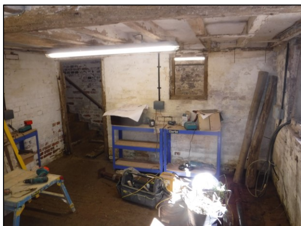
North wall of Cellar
