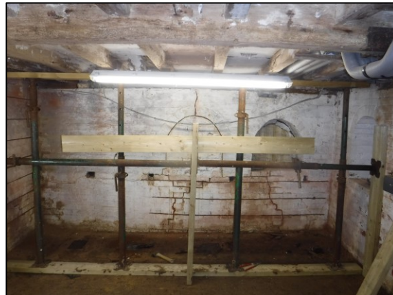
South wall of Cellar
