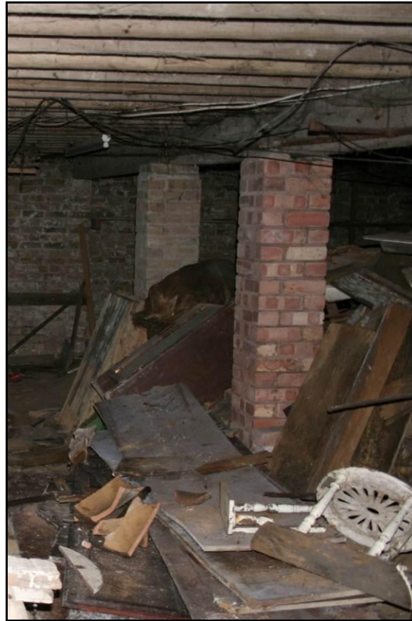
Plate 6: 28 South Way, Newhaven: Brick built pillars in basement
