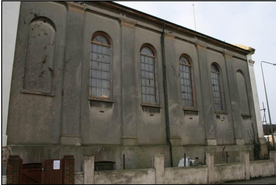
Plate 1: 28 South Way, Newhaven: Eastern Elevation
