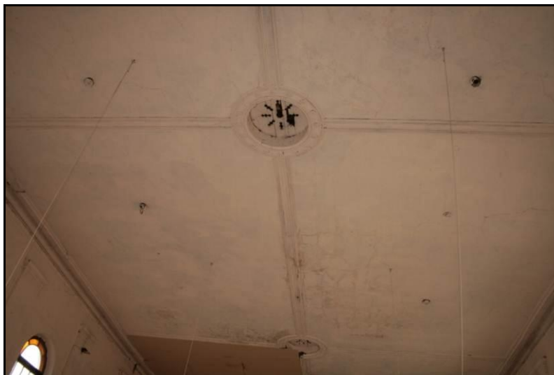
Plate 2: 28 South Way, Newhaven: The ceiling
