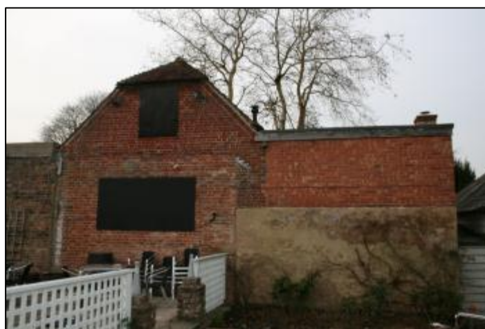
Plate 3 Tower House Eastern Elevation
