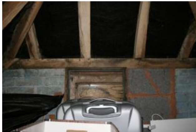
Plate 12 Tower House Windows in East Wall
