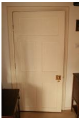
Plate 5 Tower House Door G2
