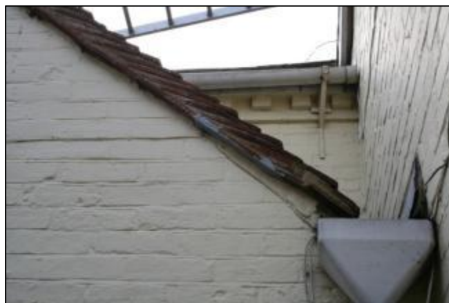
Plate 4 Tower House North wall of original house
