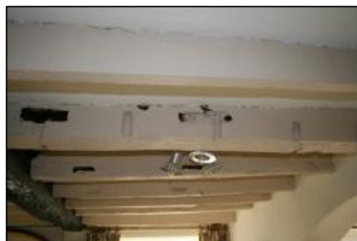
Plate 8 Tower House Possible stave holes G2
