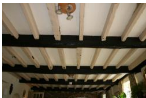
Plate 7 Tower House Ceiling in G2
