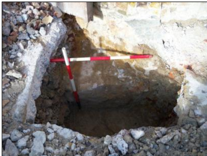
Plate 7: South facing section showing Counter Scarp Wall foundation
