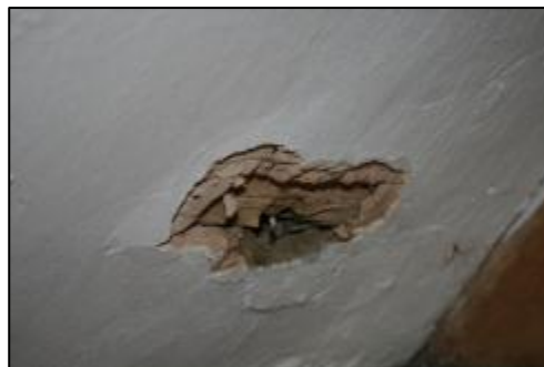
Plate 5: St Margarets Lathes and plaster
