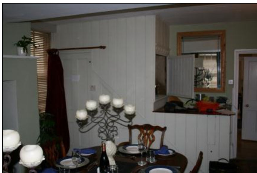
Plate 3: St Margarets The boxed-in staircase
