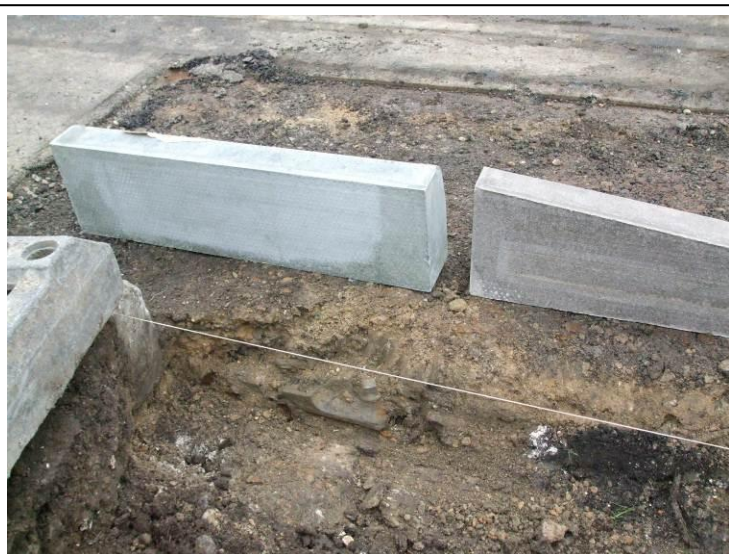
Plate 3: Detail of intact Sleeper and Rail Chair found at the junction with Ringwood Road (Chain 0.0)
