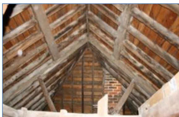
Plate 12: 224 High Street: Eastern Roof Truss
