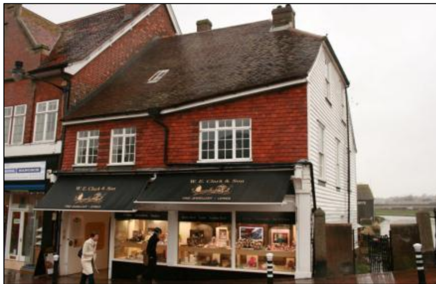
Plate 2: 224 High Street: Southern Elevation
