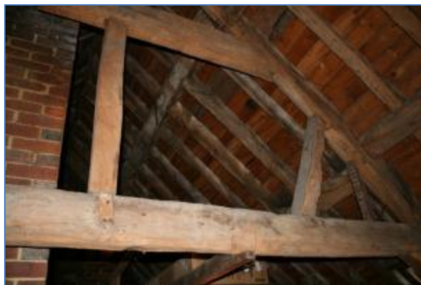
Plate 11: 224 High Street: Western Roof Truss
