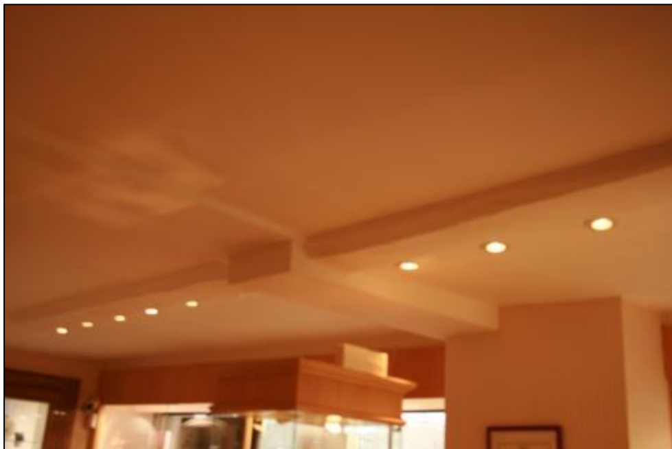
Plate 3 224 High Street Wooden beam in shop (G1)
