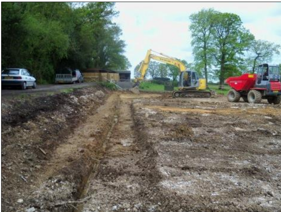
Plate 4: Plumpton Sandschool: Site during second ground reduction strip, showing drainage ditch; looking west
