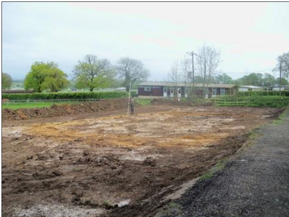
Plate 2: Plumpton Sandschool: Site after topsoil stripping, showing equestrian arena; looking northeast
