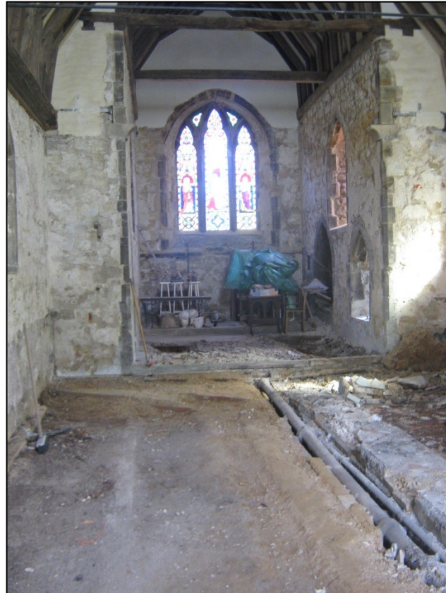
Plate 1: The interior of the church prior to any excavation work
