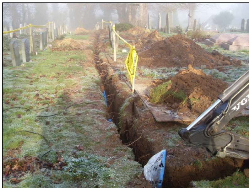
Plate 2: Service trench being excavated during the watching brief
