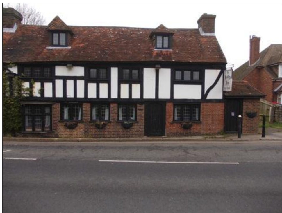
Plate 4: The Former Bridge Inn Car Park: The modified 19 th century building of The Bridge Inn, looking northeast
