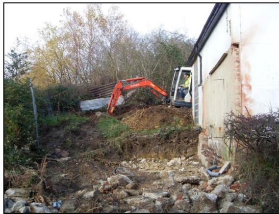
Plate 1: Excavation of topsoil and subsoil to rear of property
