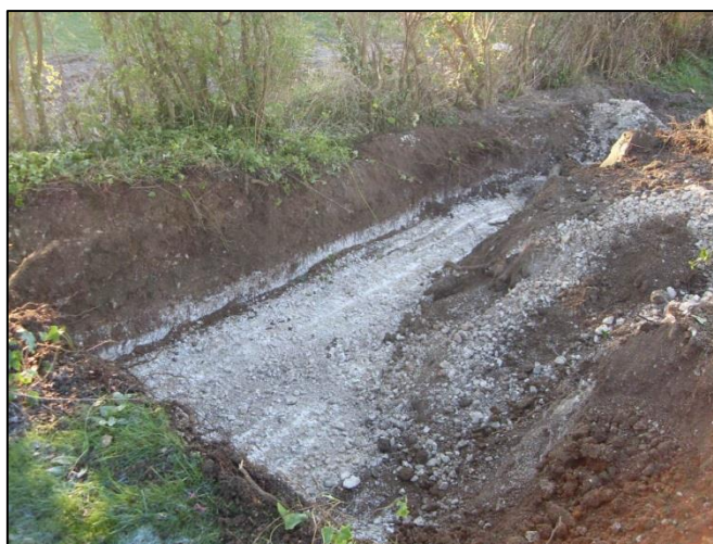
Plate 1: Excavation of house footprint
