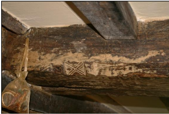
Plate 9: Saltire Design on Central Girder
