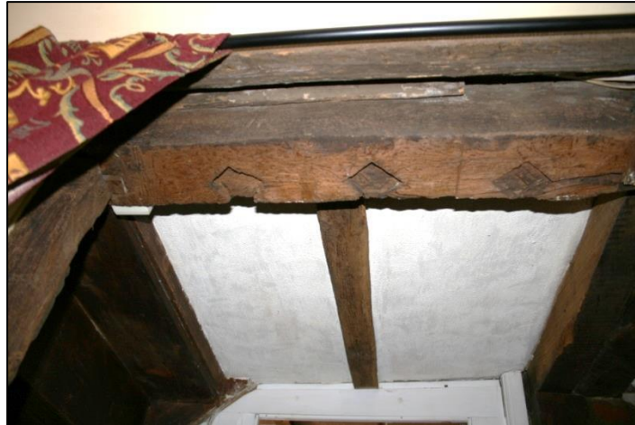
Plate 11 Diamond Shape Mortices for Window Mullions
