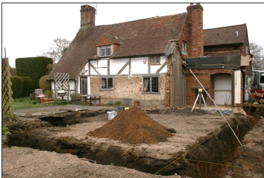
Plate 20: The Completed Footing Trenches
