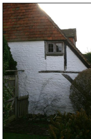
Plate 3: Sloping Timber on North Wall of Outshot
