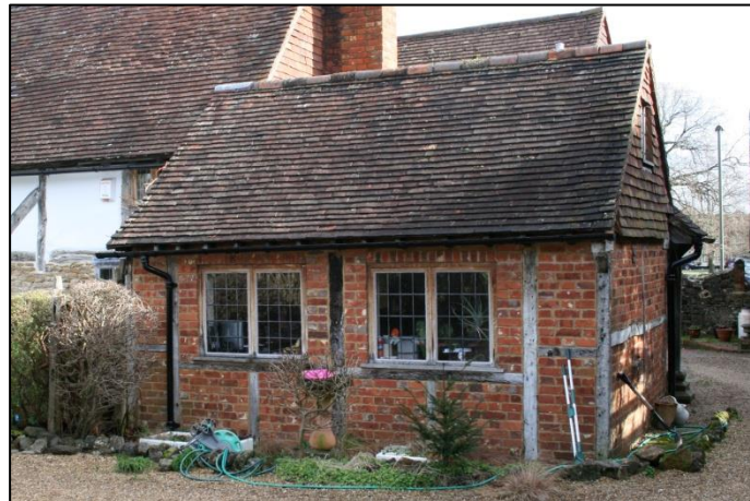
Plate 6: South-western Corner Kitchen Extensions
