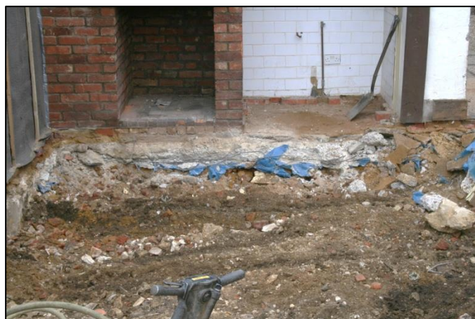
Plate 18: Concrete Floor of the 1993 Extension.
