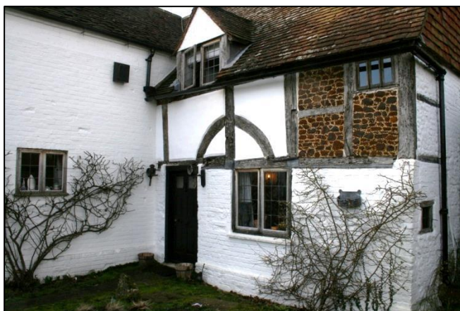
Plate 1: The Eastern Elevation of the Original Cottage
