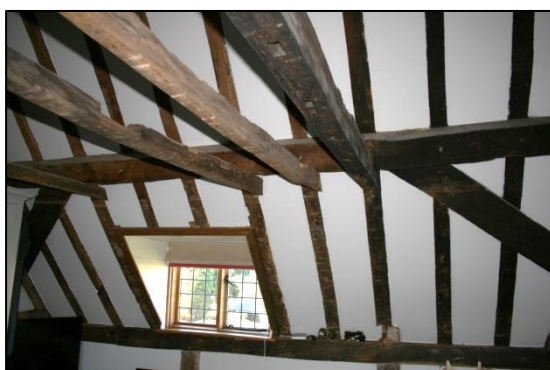
Plate 16: Wind braces Western Side
