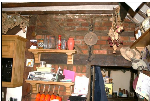
Plate 12: The Timber framing in The 1993 Kitchen Extension
