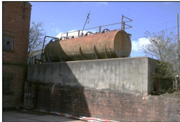
Plate 1: Building A Cylindrical Tank
