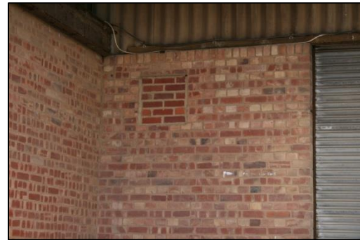
Plate 5: Building A Repair in Recessed Southern Wall
