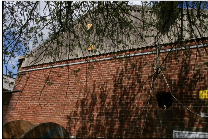
Plate 16: Building B Southern Elevation
