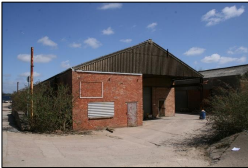
Plate 4: Building A Southern Elevation
