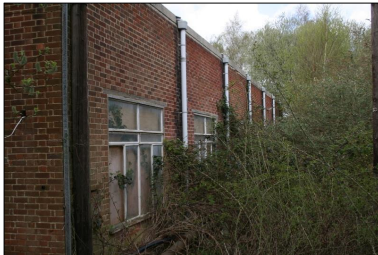
Plate 17: Building B Eastern Elevation
