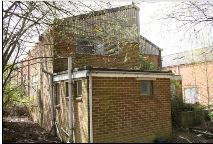
Plate 14: Building B Northern Elevation
