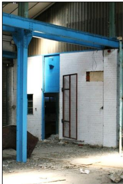
Plate 13: Building A Metal grille
