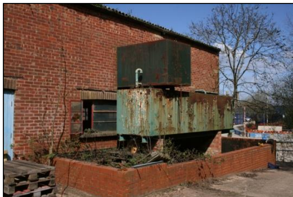
Plate 8: Building A Tanks Adjacent North End of Eastern Elevation
