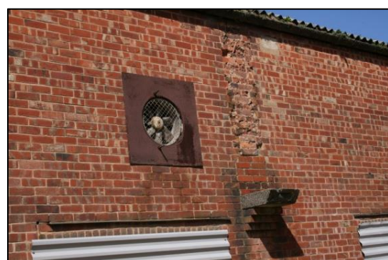
Plate 7: Building A Corbel and Ventilator
