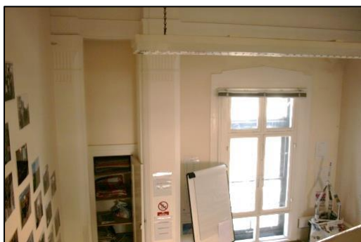
Plate 29: Paired Pilasters on North Wall of C10
