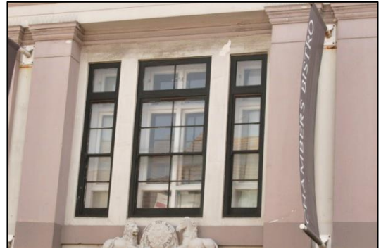
Plate 4: Original Windows behind the New
