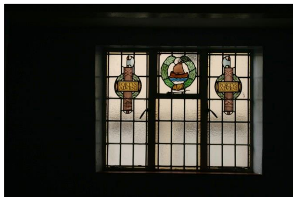
Plate 18: Window in Lower South Wall
