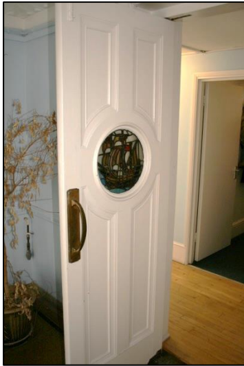
Plate 15: First Floor Landing Doors
