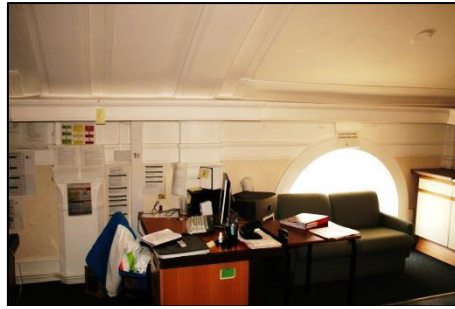
Plate 31: Top of Pilasters D2
