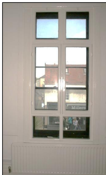
Plate 21: Example of Window in North Wall of C1
