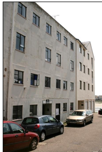
Plate 6: Western Elevation of The Annex
