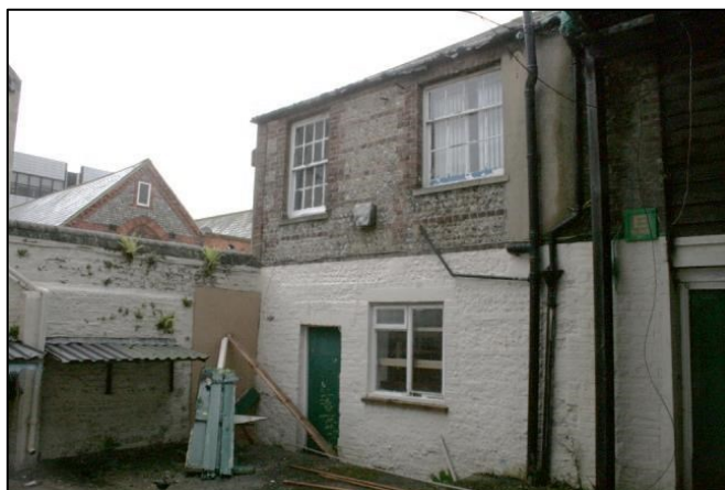
Plate 39: Northern Elevation of 89 Portland Road
