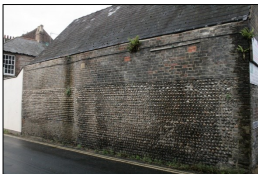
Plate 12: Eastern Elevation of Building B
