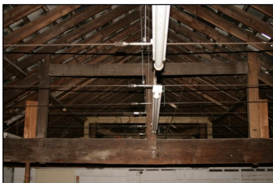
Plate 31: Eastern Trusses C2
