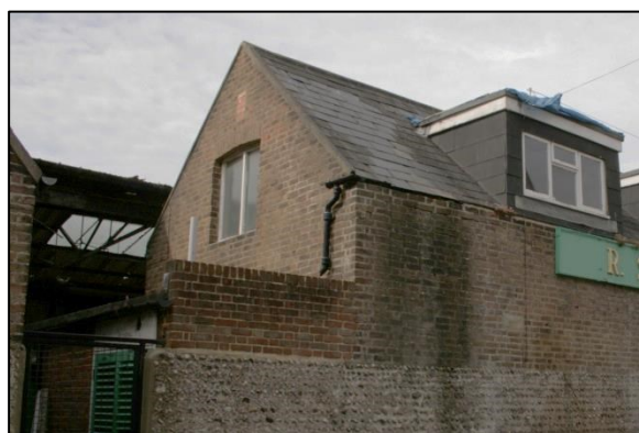
Plate 5: Eastern Elevation Building A
