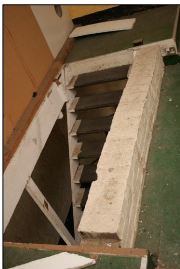
Plate 63: Top of Southern Wall of Staircase D7
