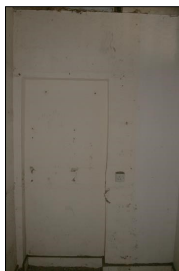
Plate 46: Sealed Doorway P3
