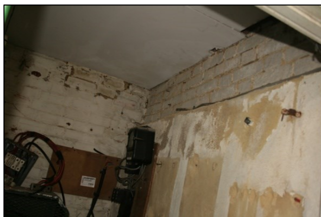
Plate 8: North Wall of the Compressor Room
