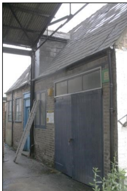
Plate 15: Projecting Structure on Roof Building B
