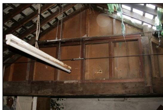
Plate 32: Western Truss C2
