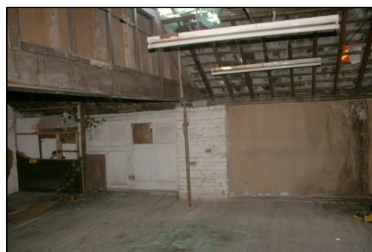
Plate 28: West End of North Wall C2
