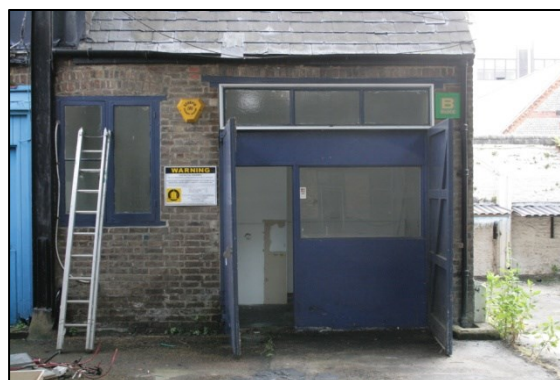
Plate 10: Security Double Doors Southern End
