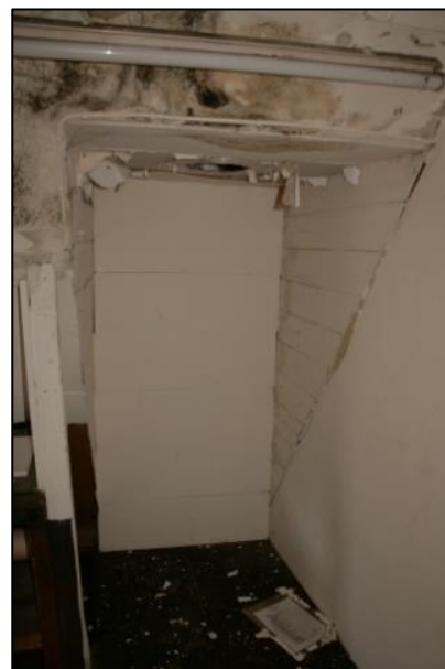
Plate 19: Projecting Gable Structure B5
