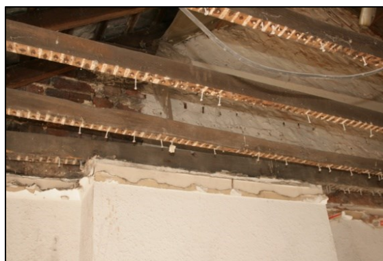
Plate 48: Ceiling Joists in P1
