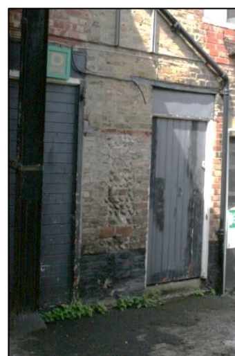
Plate 54: Panel of Flintwork
