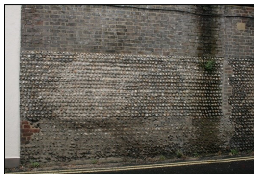
Plate 13: Southern end of East Wall Building B
