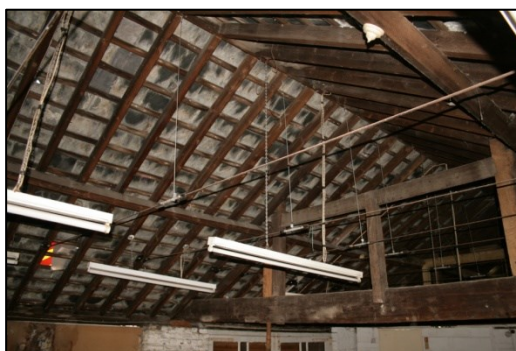
Plate 68: Continuous Roof Structure over Buildings C and E
