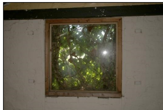
Plate 65: Window in South Wall D8
