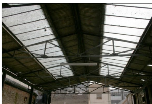
Plate 67: Six English Trusses in Canopy
