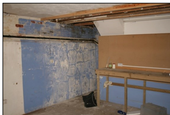
Plate 7: North and East Walls of A2
