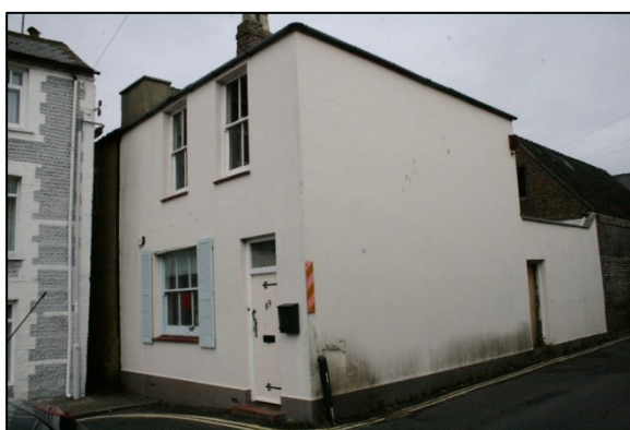
Plate 40: Eastern and Southern Elevations of 89
