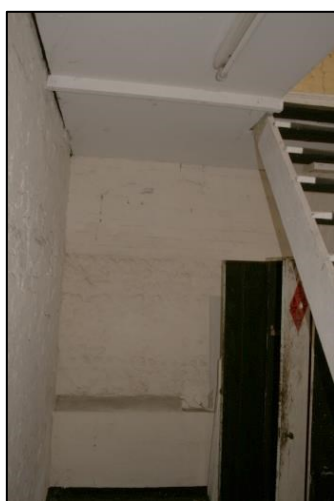
Plate 57: Western Wall D3
