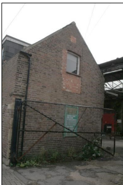
Plate 2: Western Elevation of Building A
