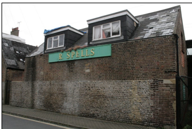
Plate 3: Northern Elevation of Building A
