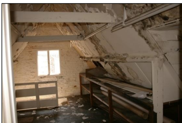
Plate 18: Visible Roof Structure B5
