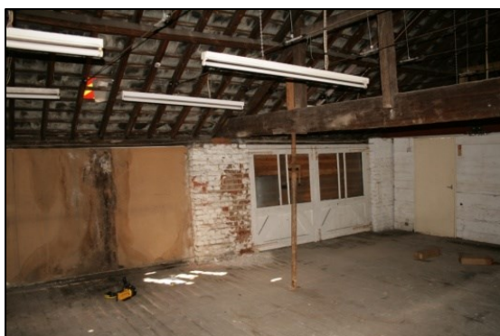
Plate 27: East End of North Wall C2
