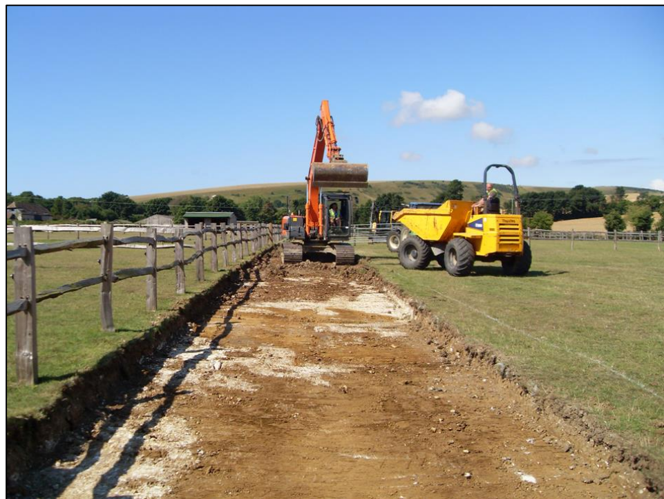
Plate 3: Working shot looking west, showing Contexts 1 to 6.
