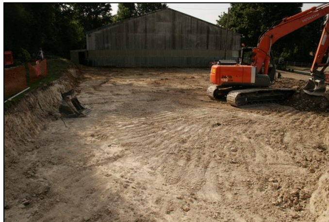
Plate 2: Ground reduction over stable block
