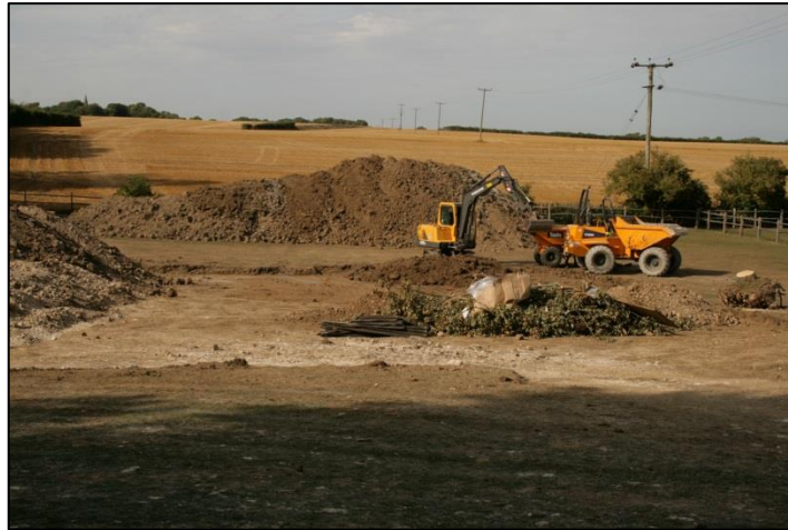
Plate 2: Removal of topsoil in the field to the north of stables
